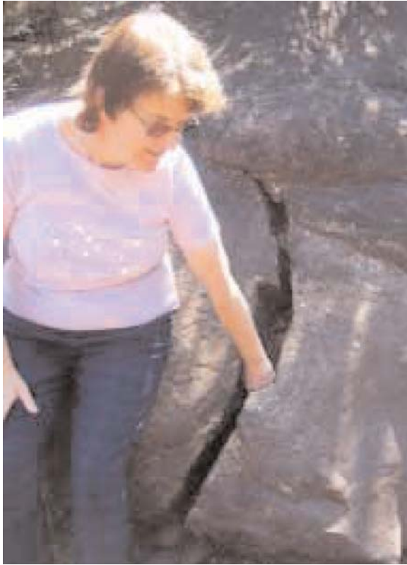
Cataract River: crack caused by longwall mining.
